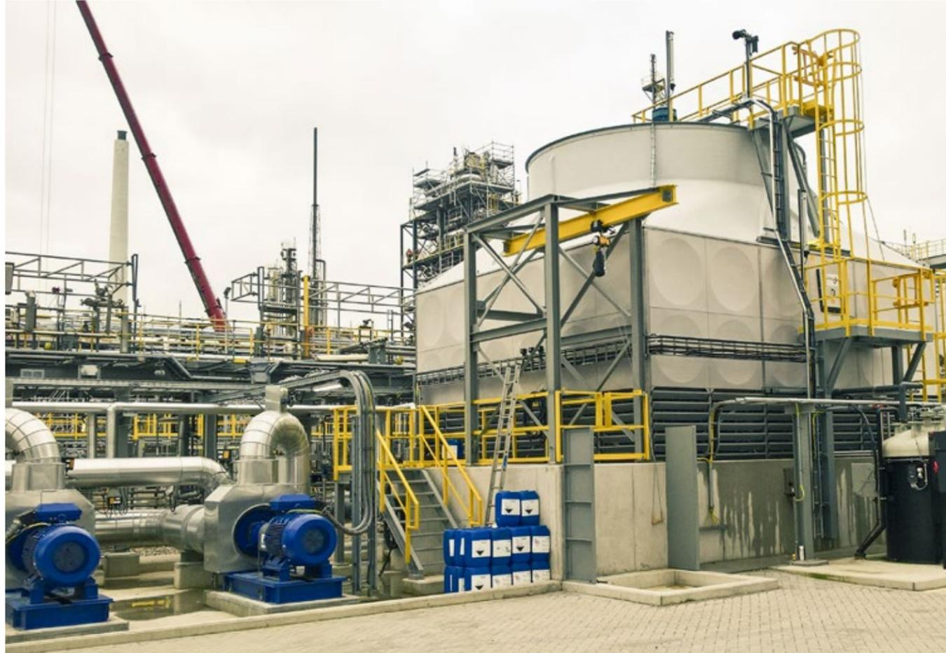
The Polacel counterflow series CMC and CMDR are characterized by a combined motor gearbox unit that is mounted directly on top of the cooling tower above the axial fan. There is a wide range of models with thermal capacities up to 30 MW per cell.
