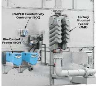
EVAPCO's **Smart Shield**<sup>®</sup> system utilizes proven solid chemistry delivered via our revolutionary feed system. Patented controlled release scale and corrosion inhibitor is fed whenever your spray water pump is energized, keeping your system protected anytime the spray water pump is operating. **Smart Shield**<sup>®</sup> is a complete water treatment package that:
