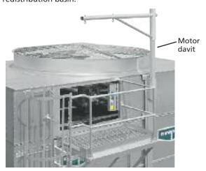
The motor davit option is an economical option which eliminates the need for a crane in the event that a fan motor has to be removed. The service mechanic needs only to have a chain-fall or come-along for easy removal of these heavy items. The motor davit is constructed from heavy duty galvanized steel with easy mounting to the unit in the field.
