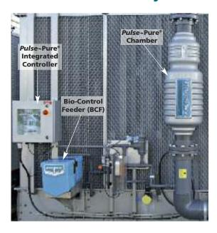
EVAPCO's *Pulse*~Pure® Plus water treatment system utilizes pulsed electric field technology to provide an environmentally responsible alternative for the treatment of water in evaporative cooled equipment. The *Pulse*~Pure® Plus system delivers short, high-frequency bursts of low energy electromagnetic fields to the recirculating water in the ESWB.
