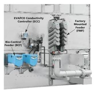
EVAPCO's **Smart Shield**® system utilizes proven solid chemistry delivered via our revolutionary feed system. Patented controlled release scale and corrosion inhibitor is fed whenever your spray water pump is energized, keeping your system protected anytime the spray water pump is operating. **Smart Shield**® is a complete water treatment package that:
