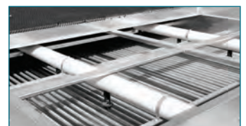
Drift Eliminators Removed for Coil Inspection
