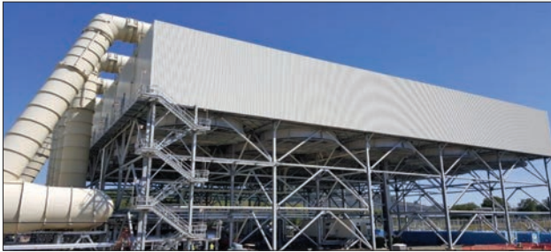
Two condensers, one structure
