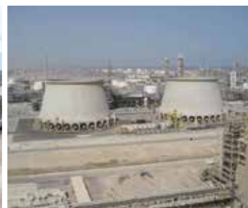
OL2K, Seawater cooling tower with an water flow of 55,000 t/h each. Kuwait
