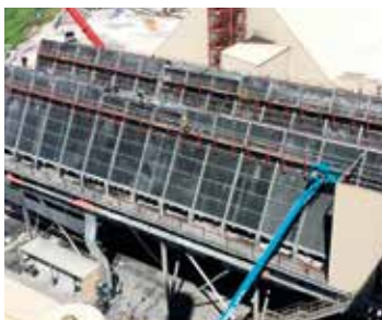
Higher cooling performance by bundle replacement
