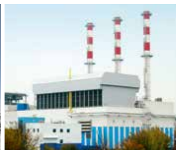
Winter proofed Mechanical Draft Heller Cooling Tower for 260 MW Co-generating CCGP, Moscow, Russia
