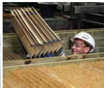
Replacement of drift eliminators and cooling fills, for example
