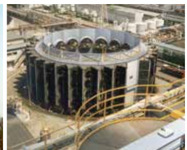
Mechanical Draft Heller Cooling Tower for a 60 MW captive power station in a Chemical plant, Japan
